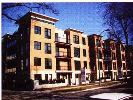
Power MBS pre-formed system erects the Sydney condo project in Vancouver for Bastion Developments.
